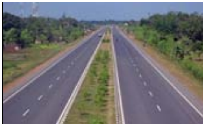
Figure 5-89 Strengthening of the NH 530B road
