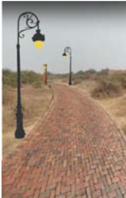
Figure 6-19: provision of brick on edge flooring to access the monuments.
