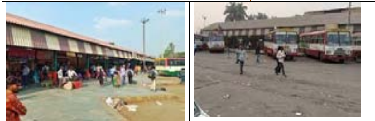
Figure 4-63: Existing condition of Satellite Bus Stand
