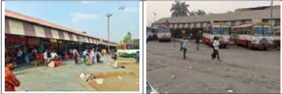
Figure 1: Existing condition of Satellite Bus Stand
