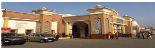
Figure 2.1.4 Bareilly Jn. Railway Station
