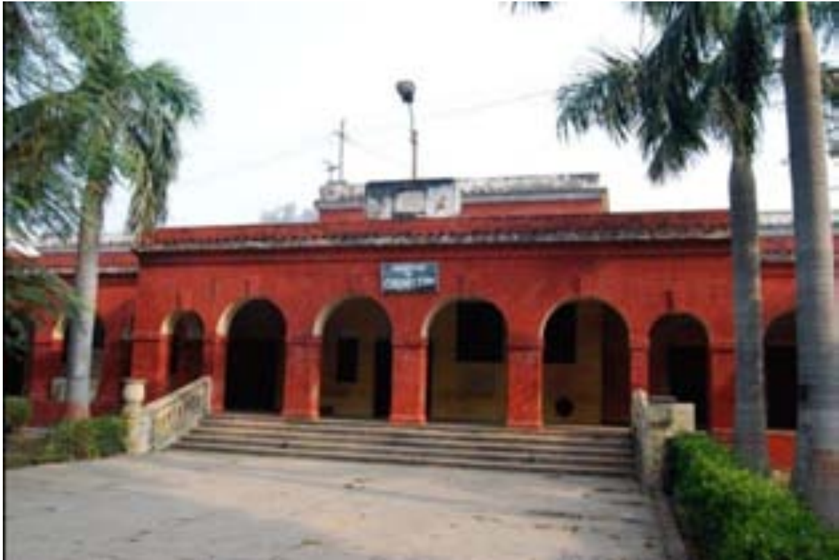
Figure 69: Current condition of chemistry department block
