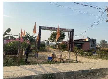
New Residential Society, G+1 Structure: Yagya Estate
