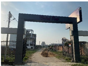
New Residential Society, G+1 Structure: Central Park
