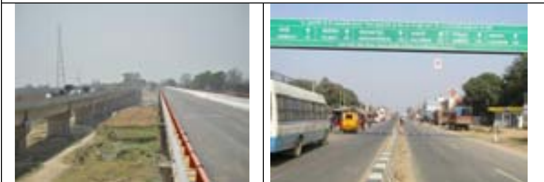
Figure 3: Major Bridge along Ramganga River
