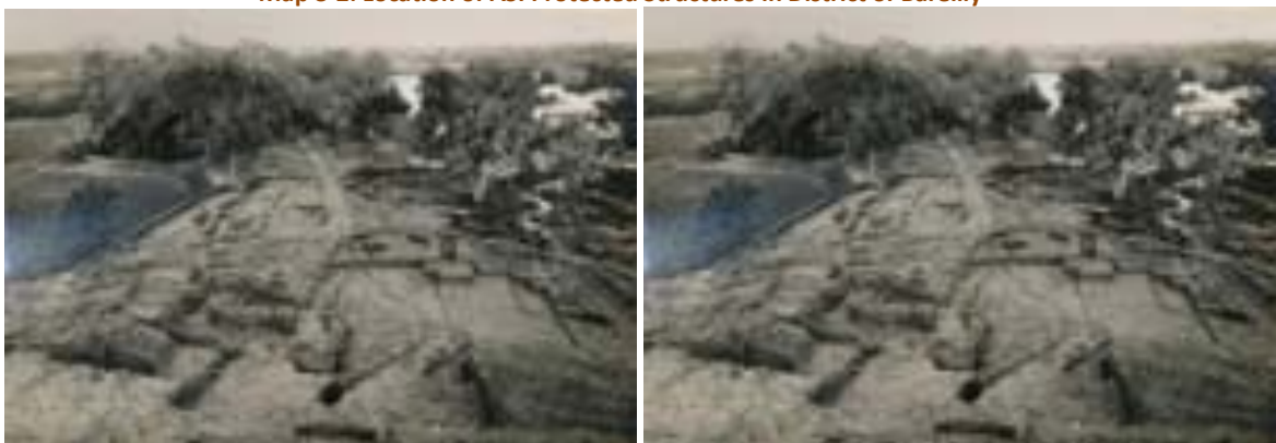
Figure 3-61: Archival image of the site excavation activities (1940-1945)
