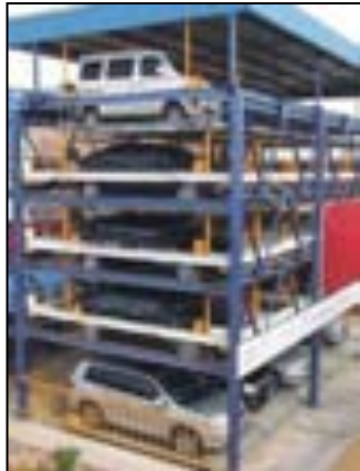
Typical Layout of Multi-level Puzzle Car parking
