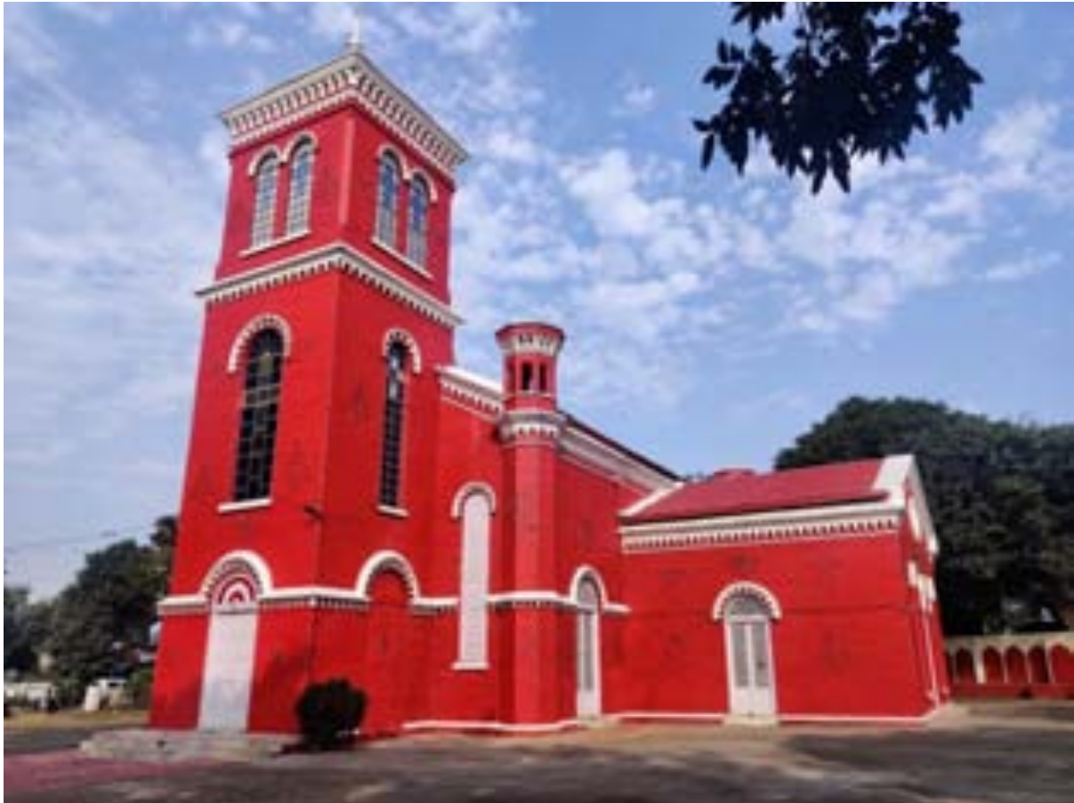
Figure 4-36 Christ Methodist Church – Civil Lines, Bareilly
