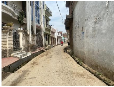
G+1 Structure: Padarathpur
