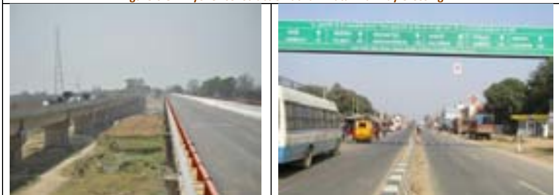
Figure 6-88: Major Bridge along Ramganga River (left) NH 530B near Binawar (right)
