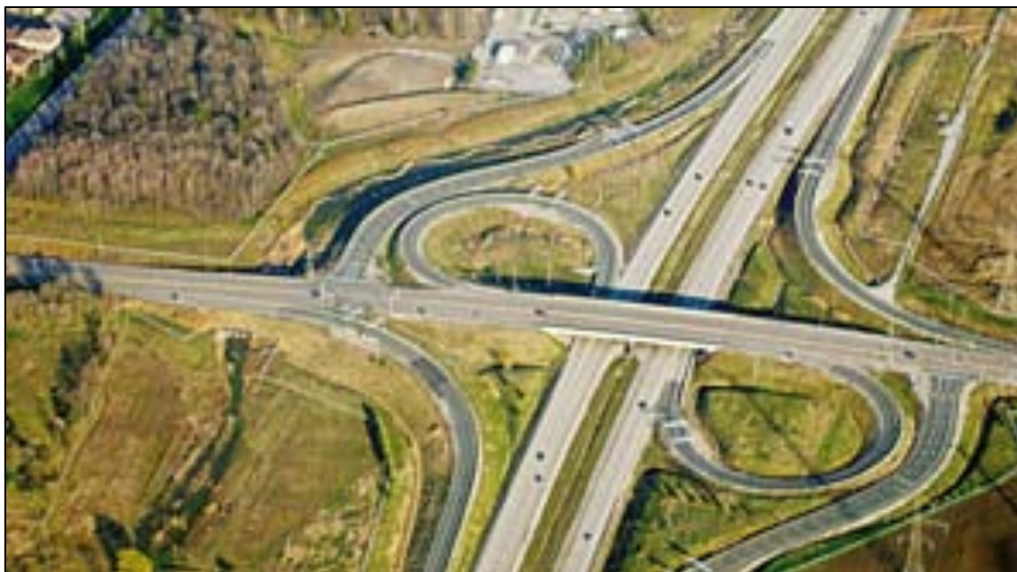
Figure 6-101: Typical layout design of Double Trumpet Interchange
