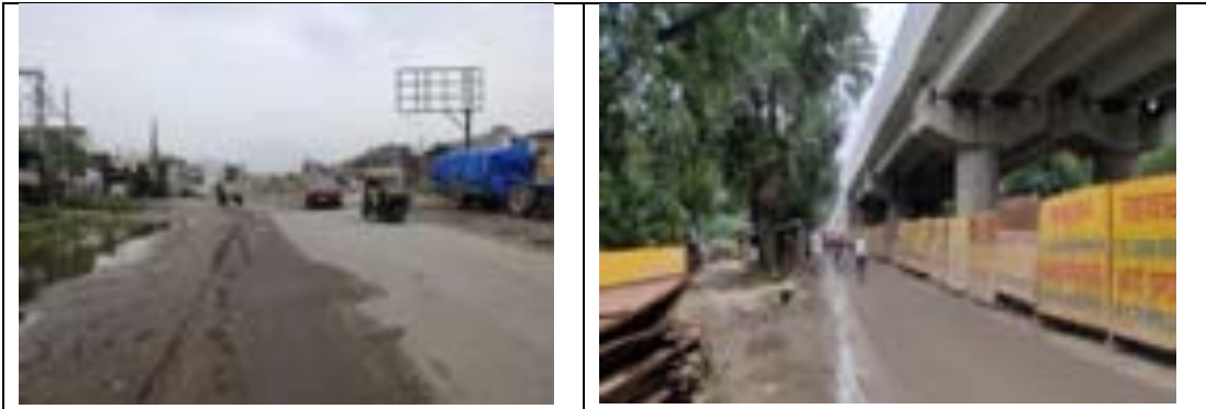
Figure 2: Flyover construction at Lal Phatak Railway Crossing
