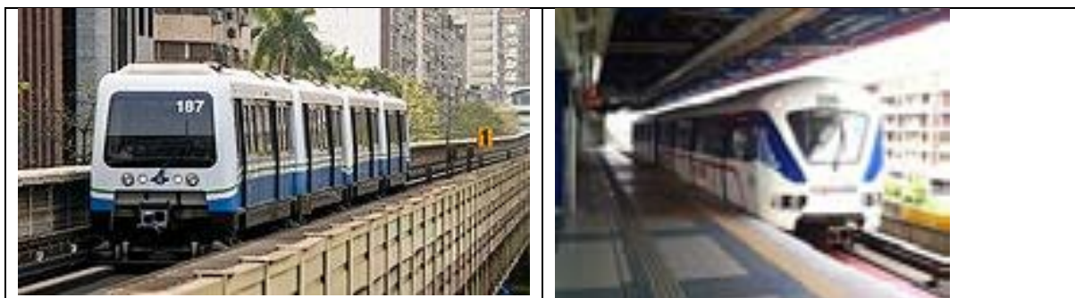
Figure 4-70: Metro light system
