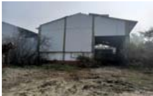
Figure 4-73: Rajau Paraspur SWM Plant
