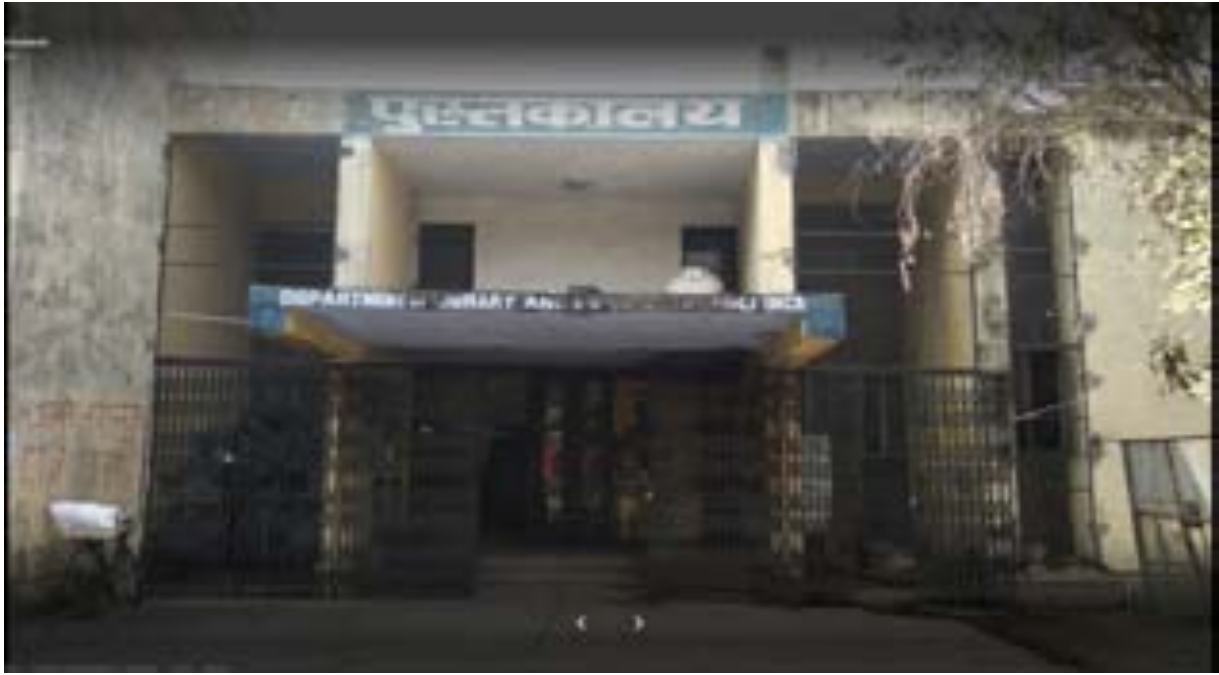
Figure 67: Image showing current condition of the library building
