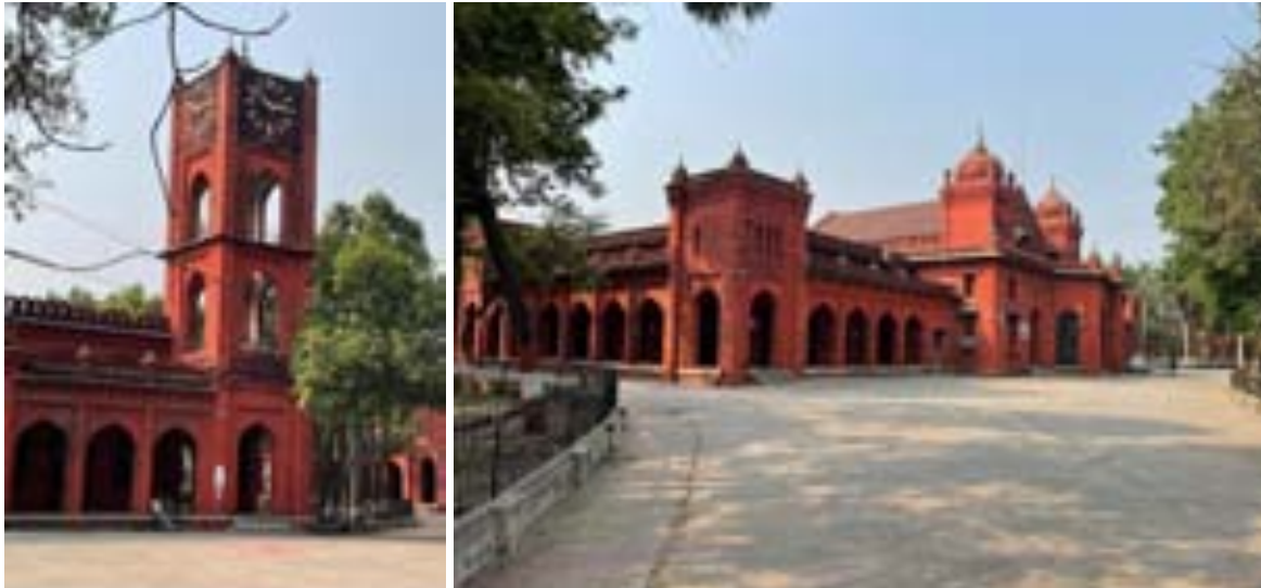
Figure 4-31 Bareilly College – Gangapur, Bareilly Source: Project Team
