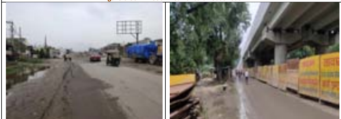
Figure 6-87: Flyover construction at Lal Phatak Railway Crossing
